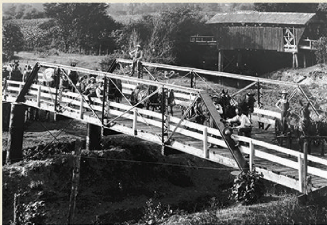
Construction of the new Rose-Dunmire Bridge in 1910. (The old 1871 covered bridge can be seen in the background.) The new iron pony truss bridge bypassed the covered bridge, as it could support larger and heavier farm equipment.
